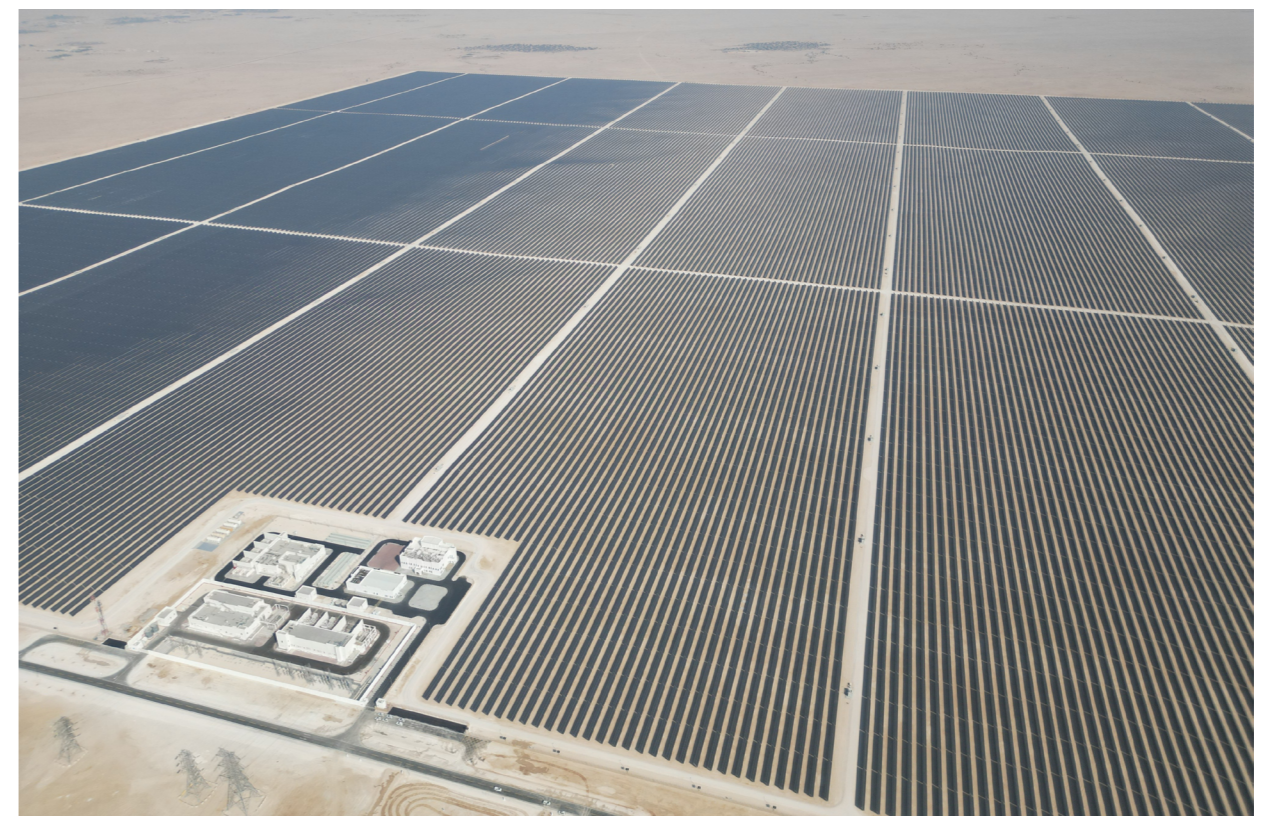
Photo of Solar Panels at Al Kharsaah Solar Plant
